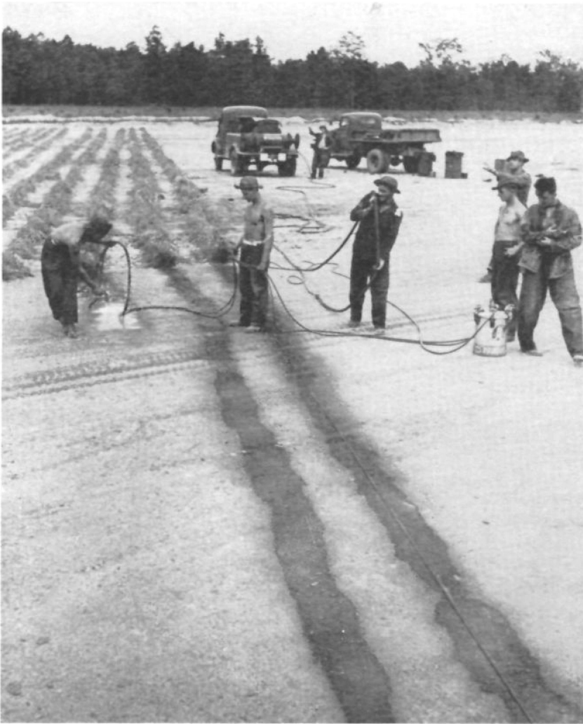
A demonstration of camouflage was staged during the maneuvers at Esler Field, Camp Beauregard. Here men of the 21st Engineers (Avn) take their simulated cabbage patch across the runway. They constructed revetments which they had intended the Blue pursuit planes stationed at the field to use. Only after the greatest persuasion could the Air Corps be induced to utilize the camouflaged facilities.
