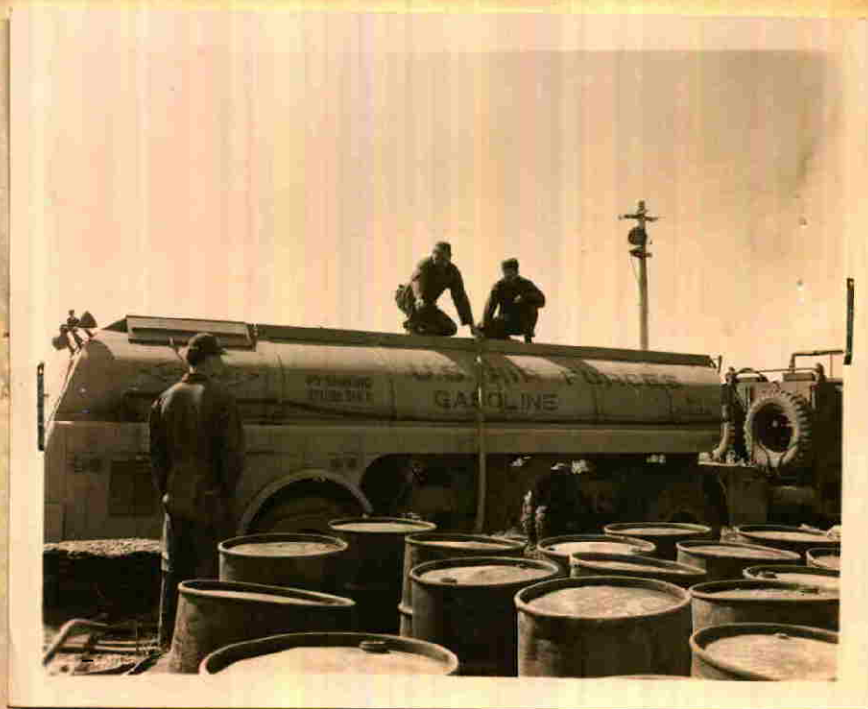
Pumping gasoline from drums into refueling trucks.
