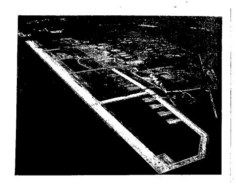
The 3,000 foot concrete strip of voloth Air dame will be a welcome improvement over the steel mat of Atsuji, but at present full operations are impossible since the publing ramp, to be located beyond the tani strip, has not yet been constructed.
